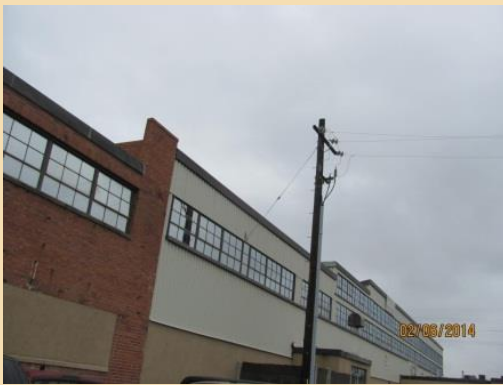
At this Location: Acceptable down guy attached to building, no marker required.
