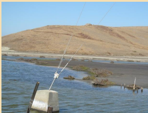
At this Location: Acceptable down guy in marsh, no marker required.
