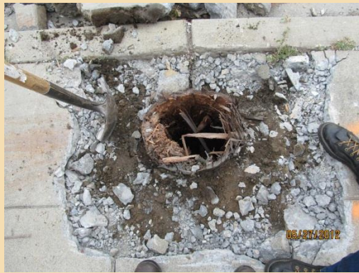
After extraction showing below ground deterioration
