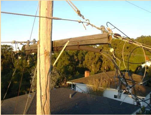
Deteriorated Crossarm
